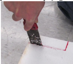
Figure 30: Cut foam insulation
